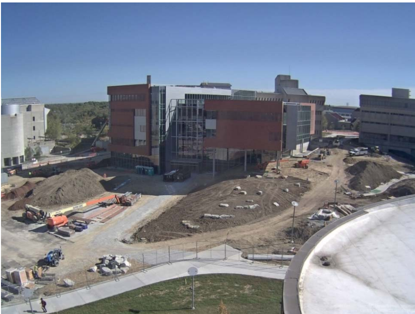
Webcam Photo of Construction Site, October 3, 2017
