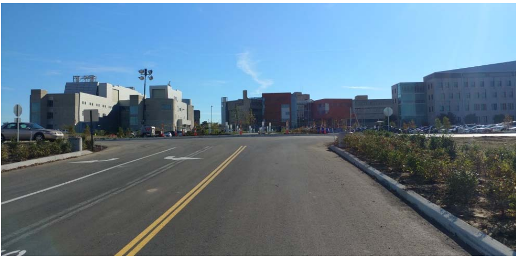
View of Lot K and Campus from Connector Road Driveway – Oct. 2
