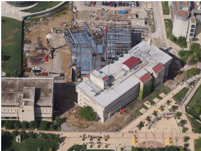
Aerial Photo of Construction Site - 2
