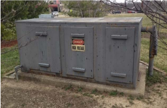
Current 'Pad Mount' Loop Switch
