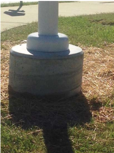
New pole base
