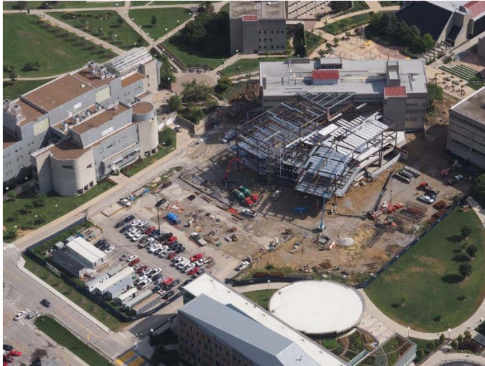
Aerial Photo of Construction Site - 1
