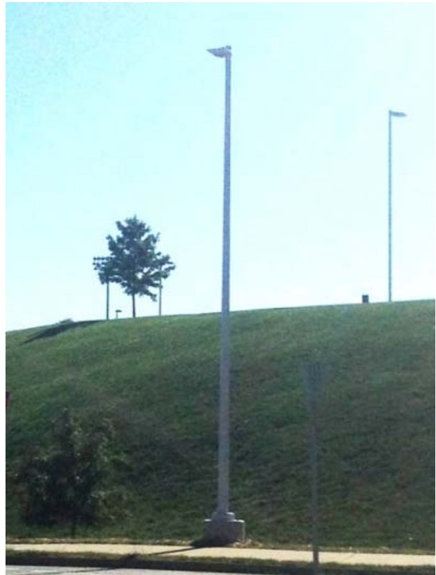
New light pole
