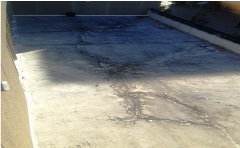
Current condition of the roof
