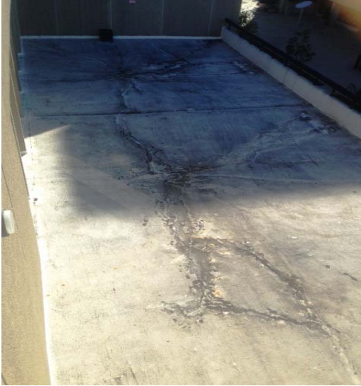
Previous Condition of the Roof
