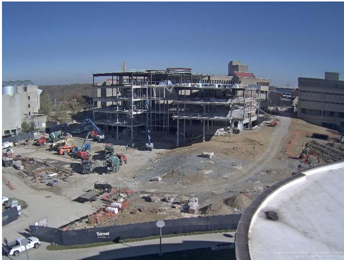
Webcam Photo of Construction Site
