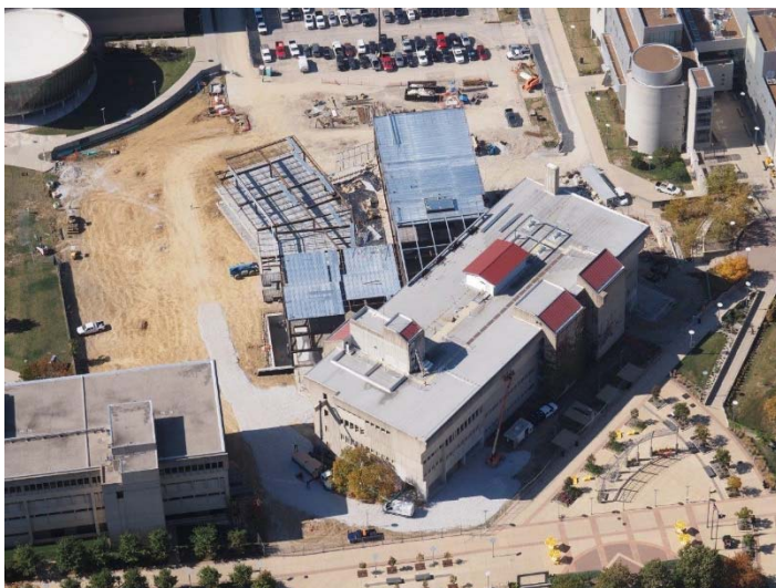
Aerial Photo of Construction Site
