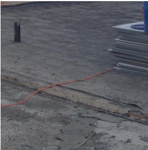
Roof Repair Work in Process
