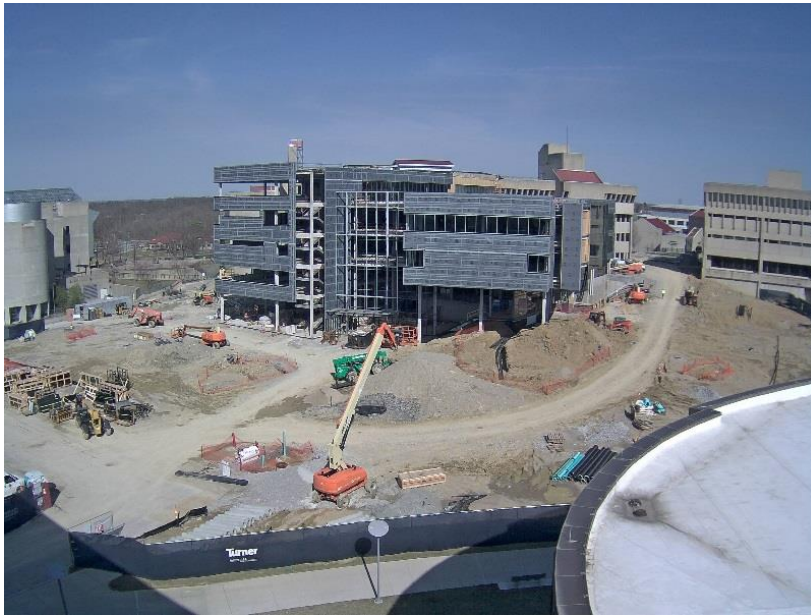
Webcam Photo of Construction Site
