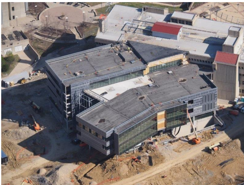
Aerial Photo of Construction Site
