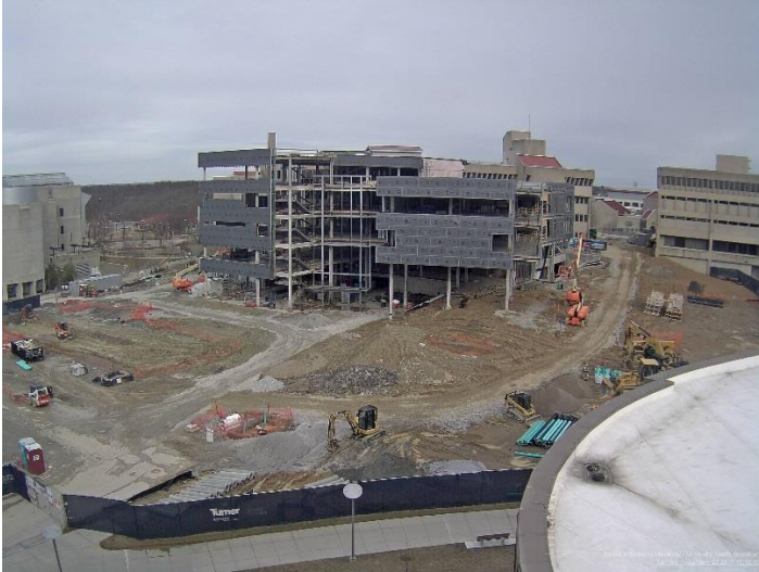
Webcam Photo of Construction Site
