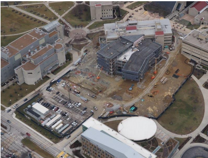
Aerial Photo of Construction Site
