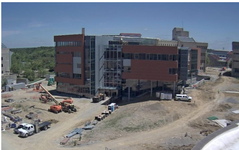
Webcam Photo of Construction Site, July 28, 2017
