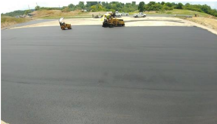
Paving of Lot A (West of Kenton Garage, with Connector Road in Background) – July 18
