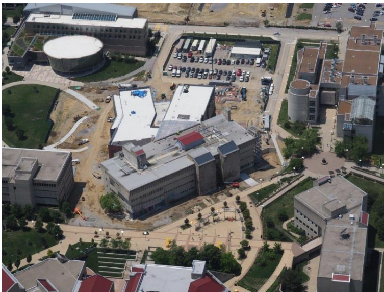
Aerial Photo of Construction Site, mid-July 2017
