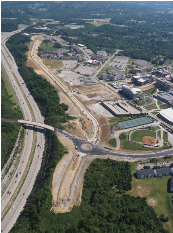
North Connector Road Aerial Photo, June 2017
