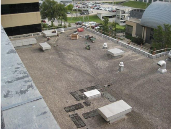
Roof condition when the project started.
