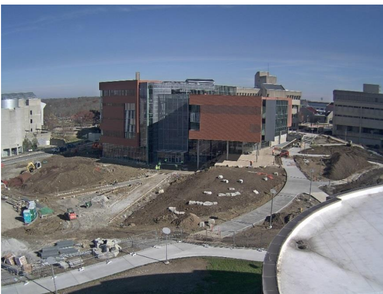
Webcam Photo of Construction Site, November 17, 2017
