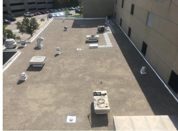
Roof condition near the end of the project
