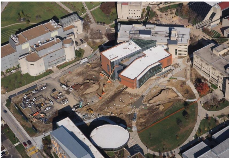
Aerial Photo of Construction Site, mid-November 2017
