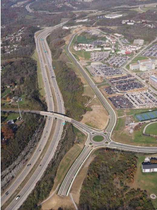
Norse Boulevard Aerial Photo, November 2017
