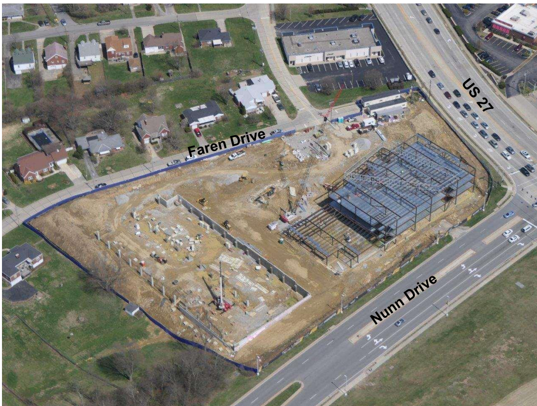
Aerial of Phase I Site as of April 1, 2019
