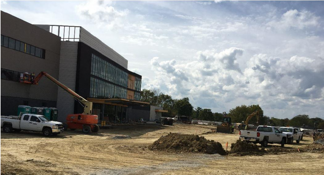
Main Entrance Site Grading – October 10, 2019
