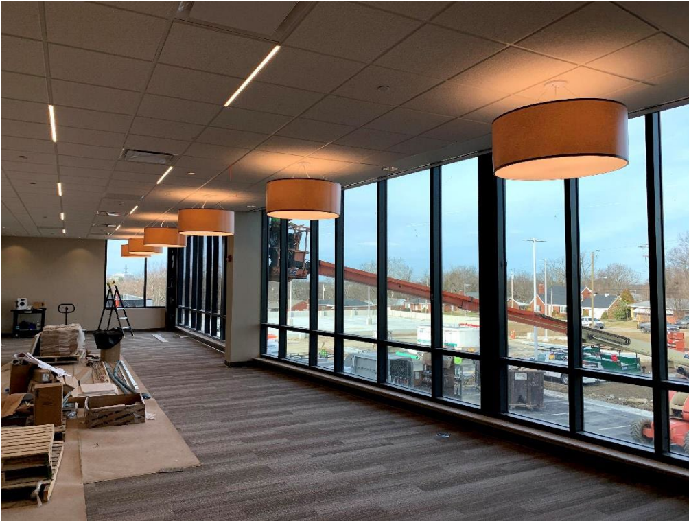
Hanging Light Fixtures, 2/3/2020
