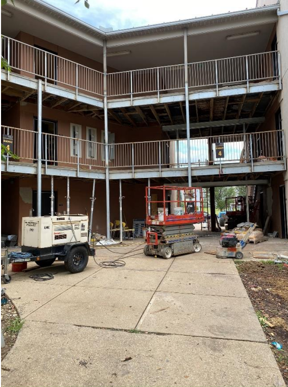
Norse Hall Balcony Railing Replacement, July 27, 2020
