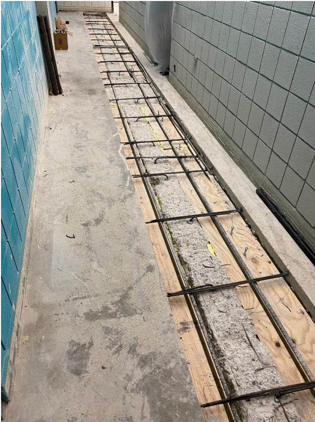
Fine Arts Center Concrete Slab Repair, Second Floor Corridor, July 2020
