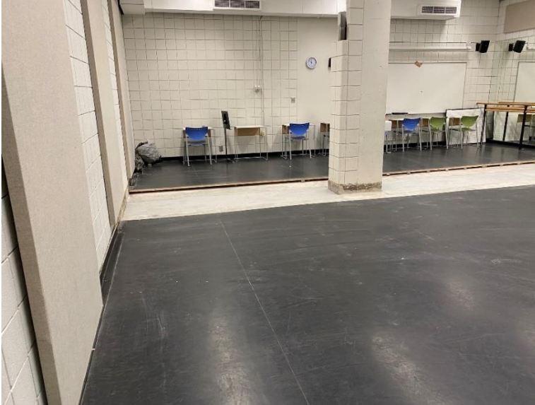
Fine Arts Center Concrete Slab Repair, FA 220 Movement Studio, July 2020
