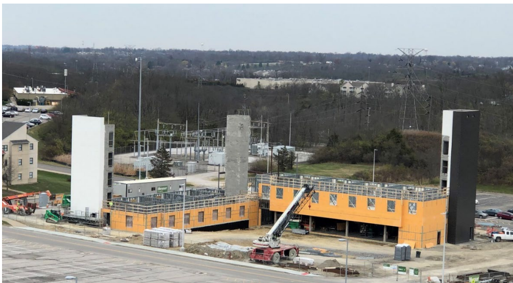
New Residence Hall (photo taken from Landrum Roof), November 2020
