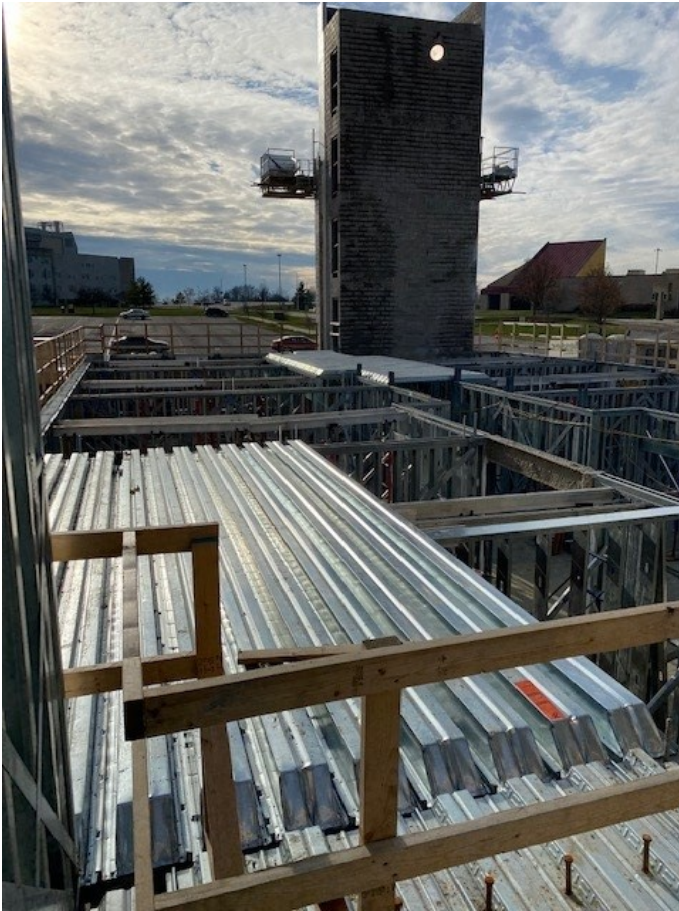
New Residence Hall Metal Decking, December 3, 2020
