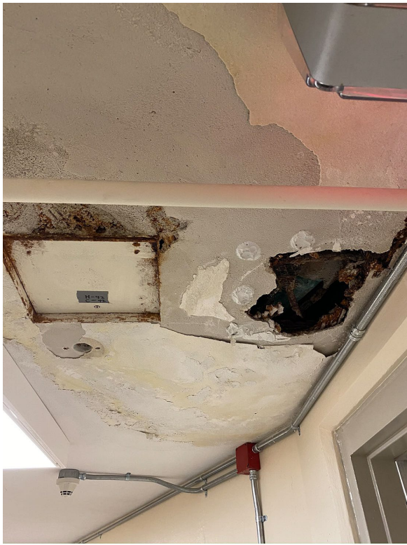
Typical basement ceiling condition due to leaks and typical mechanical closet condition.
