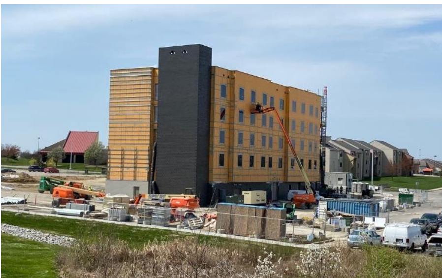
View Looking West Toward Boothe Village
