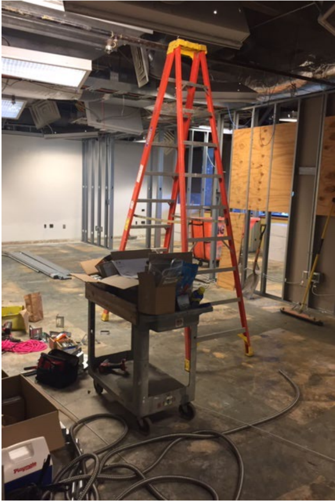
BC 243 Renovation Underway, July 30, 2021
