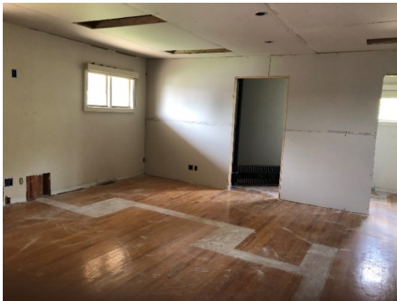
Upper Level, Dispatch Office, July 30, 2021
