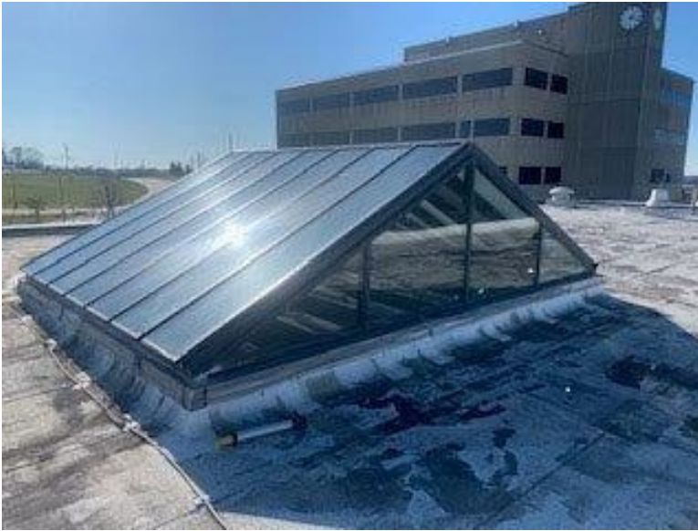
One of two existing skylights that will be replaced.
