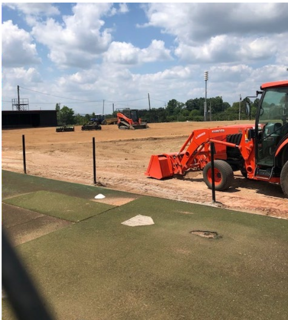
Softball Field Construction Underway
