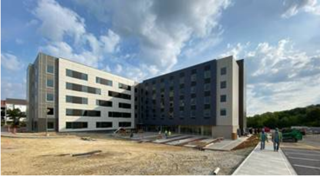
View from Carroll Drive Looking North into the Courtyard
