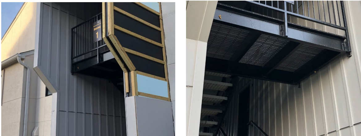
Siding Installation in Process, Norse Hall Breezeways, November 30, 2021
