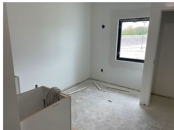
Interior of Typical Residential Unit
