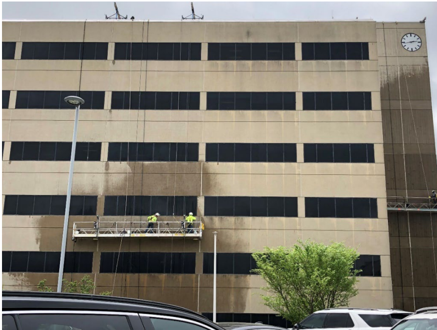
Façade Cleaning Underway, May 2022
