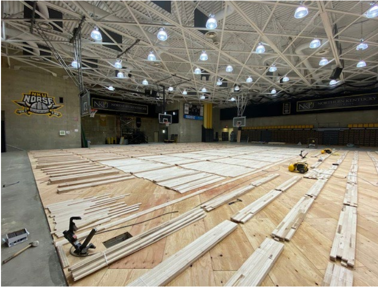
New Playing Floor at Regents Hall, May 8, 2023 Progress Photo
