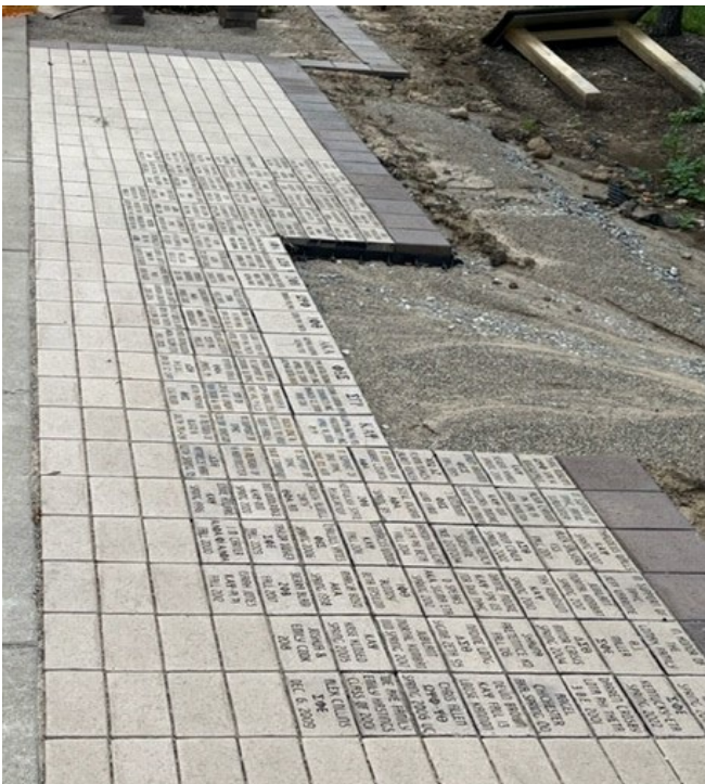
Newly installed pavers
