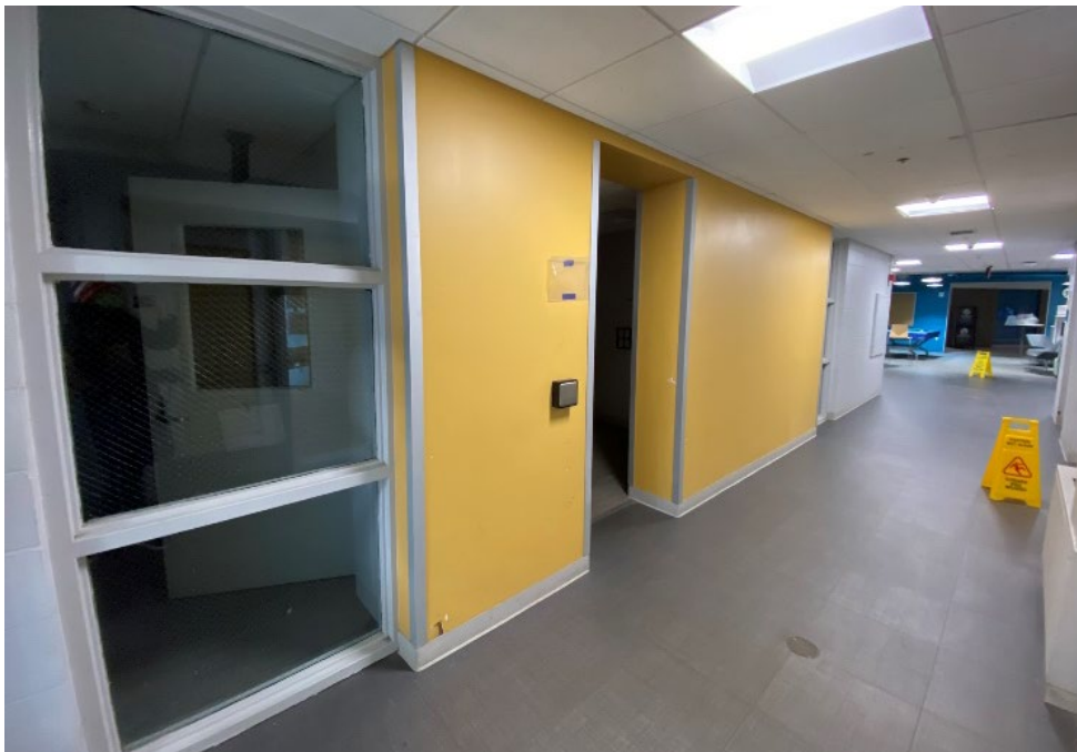
H-Wing Corridor Prior to Start of Renovation
