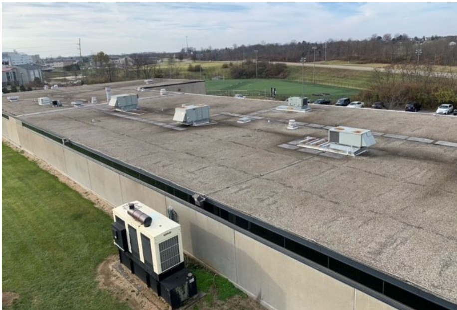
Maintenance Building Roof – November 2022
