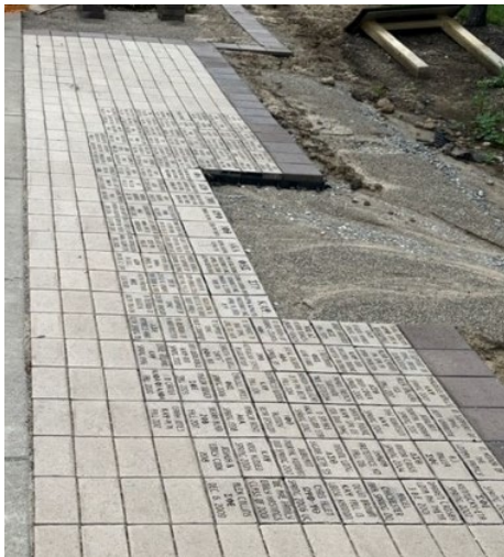
Newly installed pavers
