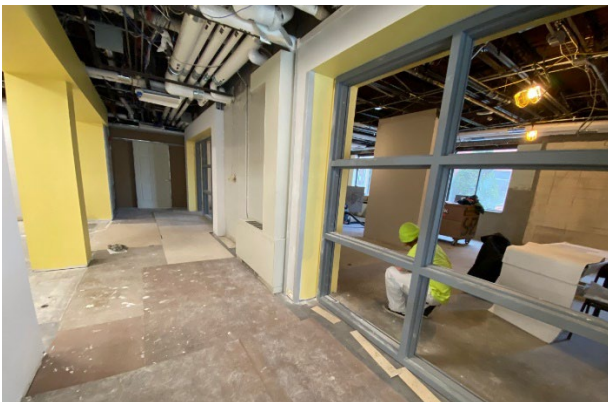
H-Wing Renovation, February 2, 2023
