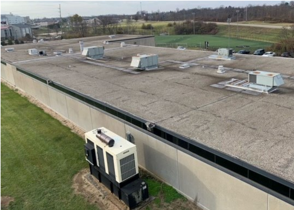
Maintenance Building Roof – November 2022
