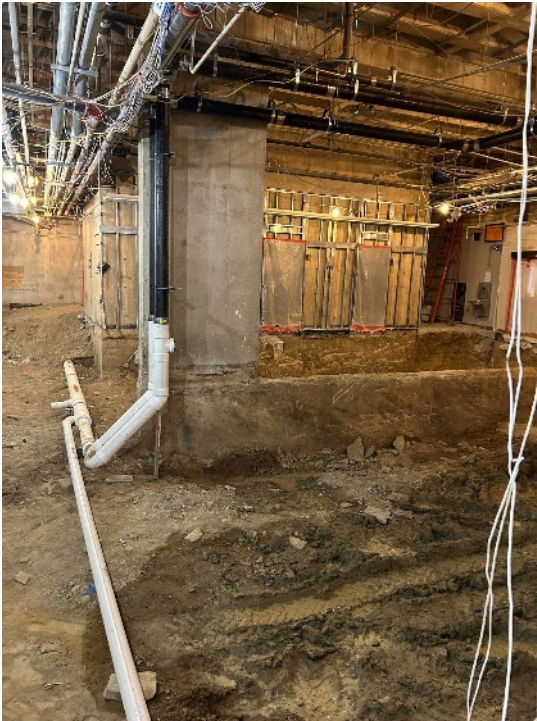
New Underground Plumbing Piping (the 1 st Floor Elevator Lobby is in the Background of this photo) and Upper Floor Restroom Renovation Underway
