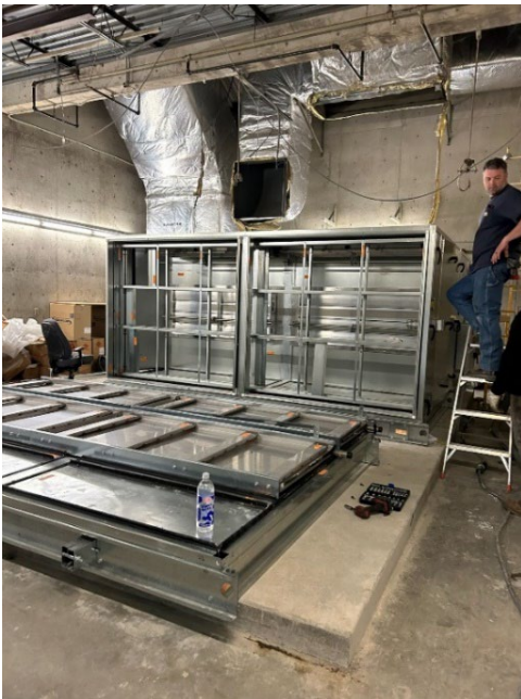
Fourth Floor Air Handling Unit Construction and New Ductwork, April 2024
