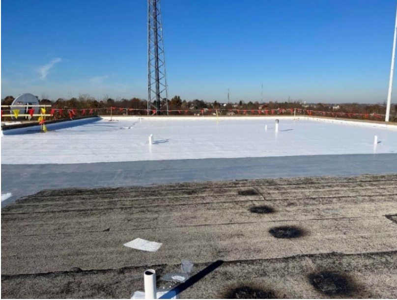
Campbell Hall Roof Restoration Underway
