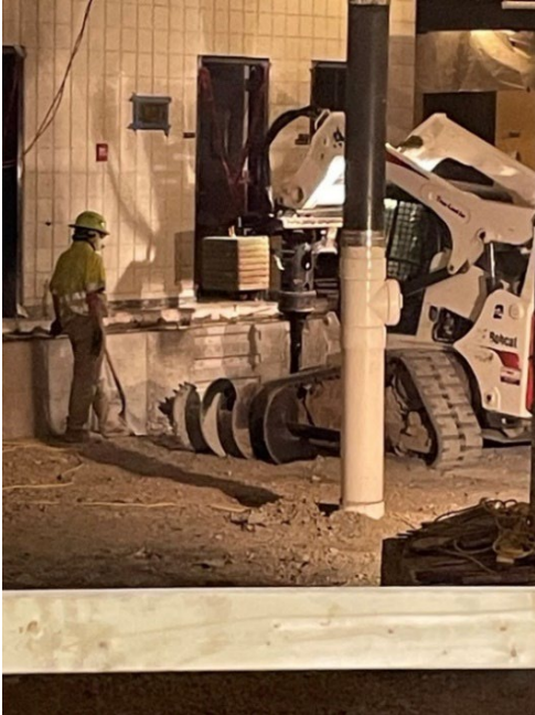
Concrete Pier and Beam Construction on First Floor, April 2024
