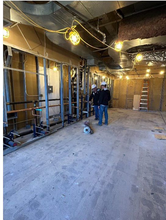
New Underground Plumbing Piping (the 1 st Floor Elevator Lobby is in the Background of this photo) and Upper Floor Restroom Renovation Underway
