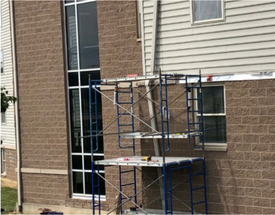
Façade Repairs Underway at University Suites
