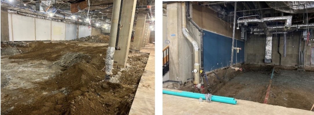
Excavation Underway in Nunn Hall
