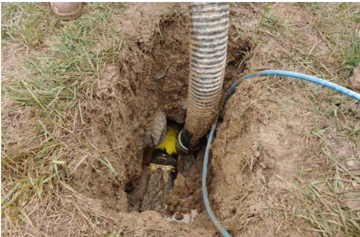
Steel and Plastic Pipe Juncture near Norse Commons
