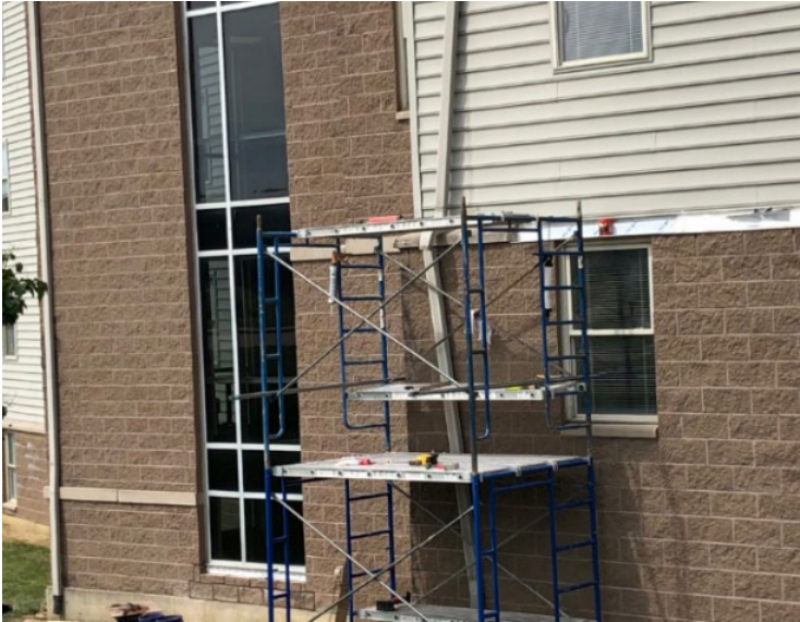
Façade Repairs Underway at University Suites
