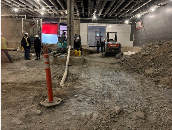
Excavation and Utility Replacement Underway in Fine Arts
