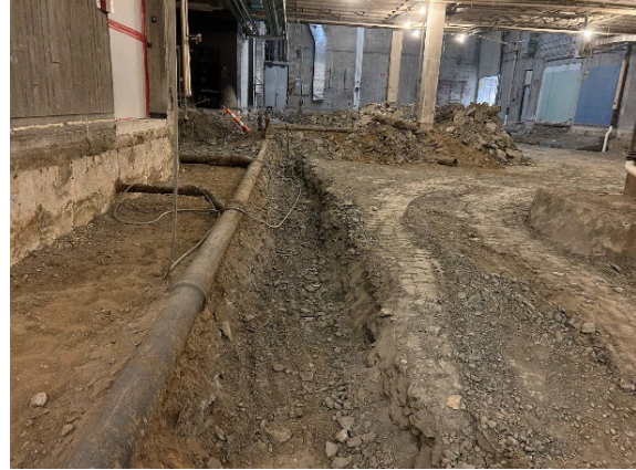
Excavation and Utility Replacement Underway in Fine Arts
