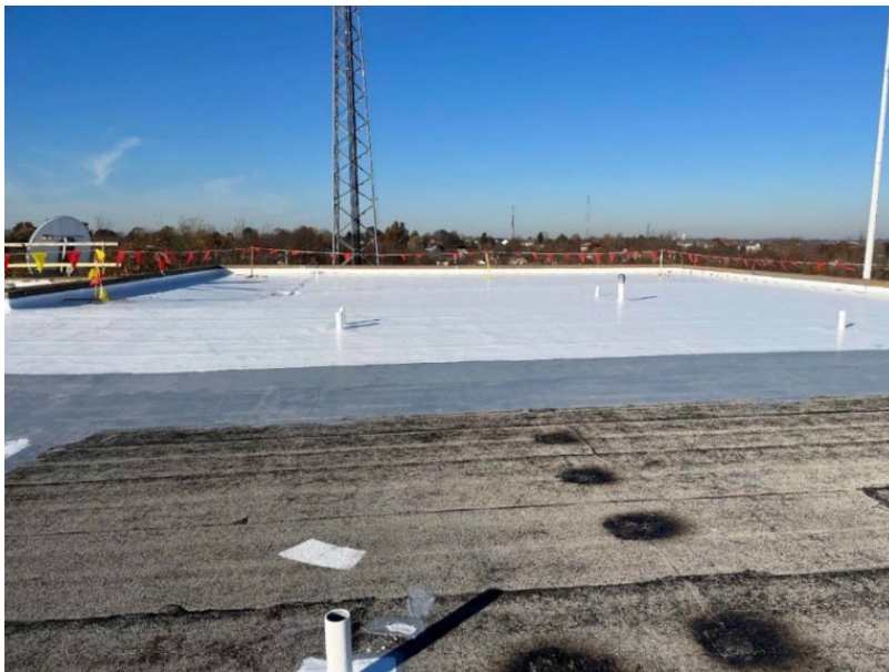
Campbell Hall Roof Restoration Underway
