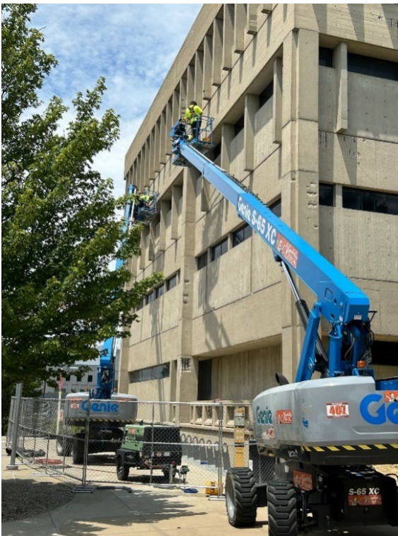
Repairs, patching and cleaning underway on Nunn Hall
