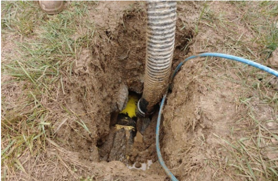
Steel and Plastic Pipe Juncture near Norse Commons
