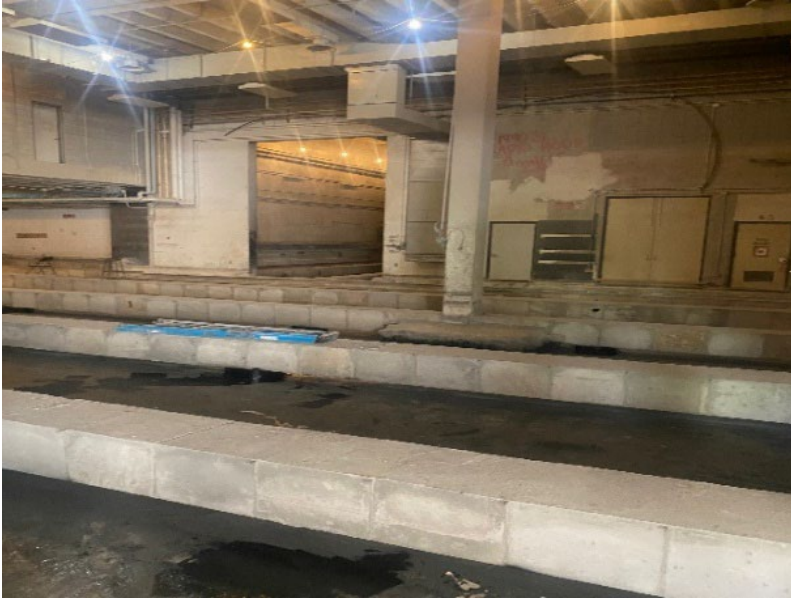
New Subfloor Structural System, July 2024
