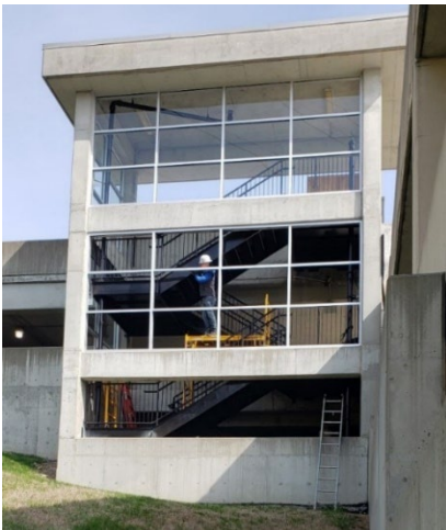
New Steel Stair and Protective Glazing
