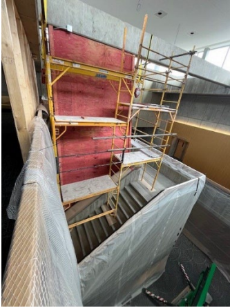
Framing for Atrium Luminaire under Construction
