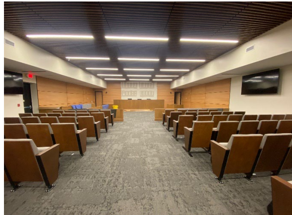
Progress Photo – New Courtroom
