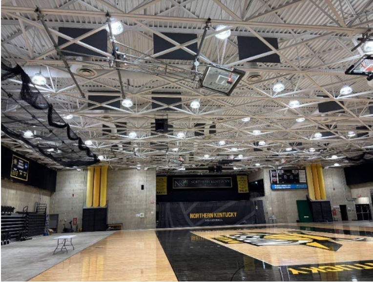
New Lighting in Regents Hall
