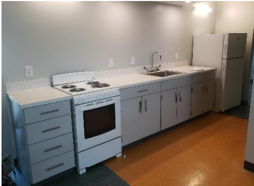
New Kitchen in Northern Terrace
