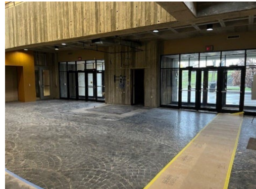
Lobby after Demolition of Bank Space
