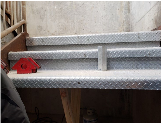
New Stair Installation in Progress
