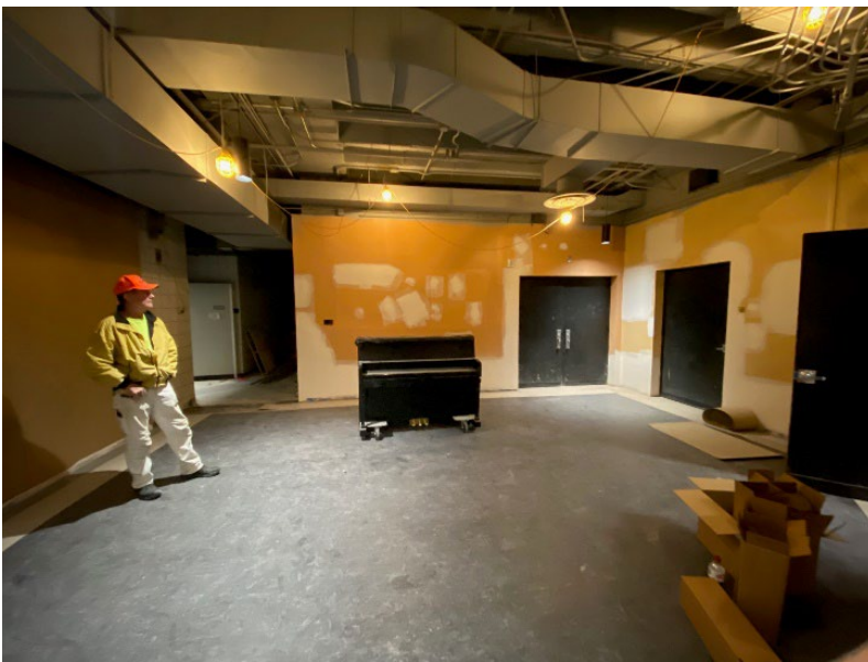
First Floor FA Elevator Lobby Looking Toward Stauss Theatre
