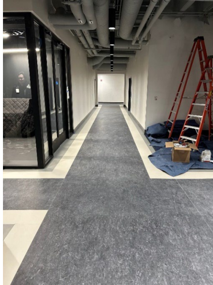
New Lobby with View of New Acting Studio
