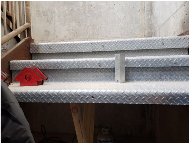
New Stair Installation in Progress
