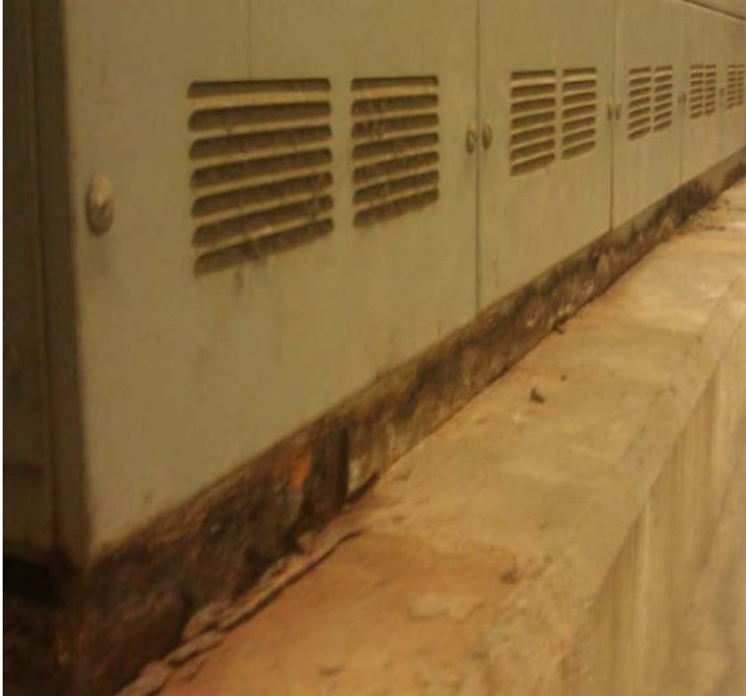
Founders Hall Switchgear before replacement
