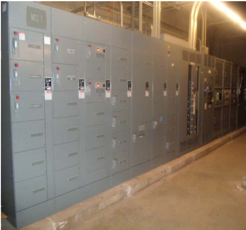
New Switchgear in Founders Hall
