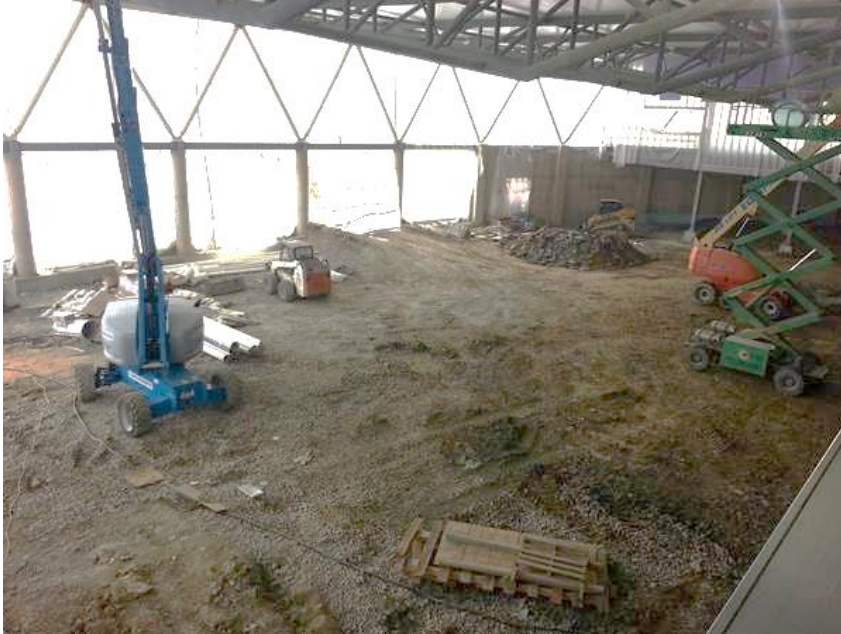
Progress Construction Photo from January 2015
