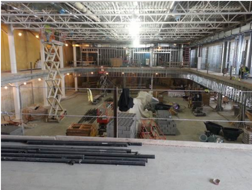
Progress Construction Photo from January 2015
