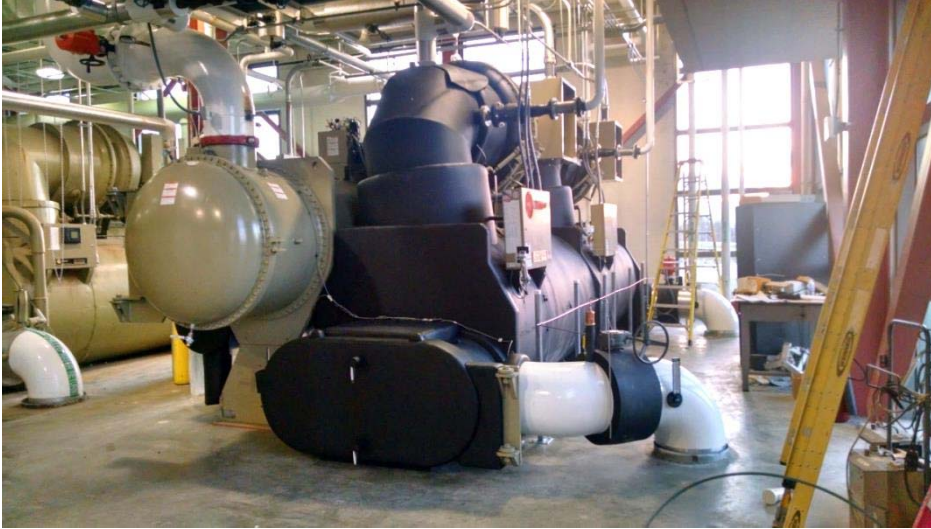
120,000 lb. Chiller being lifted into the Power Plant
