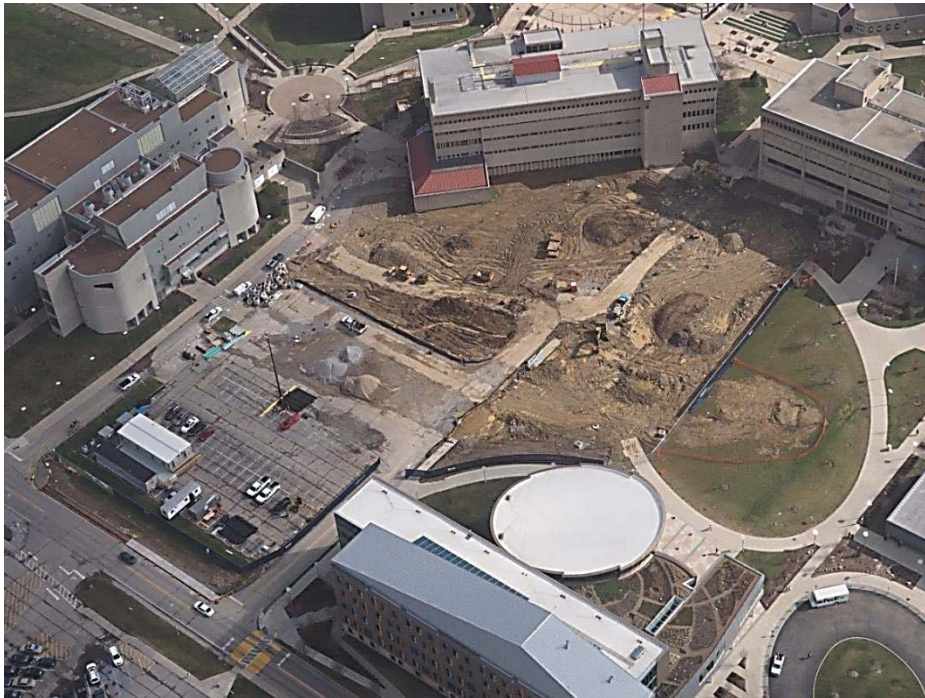
Aerial Photo of Construction Site
