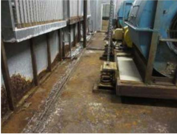
Previous condition of the Air Handlers and Mechanical Room
