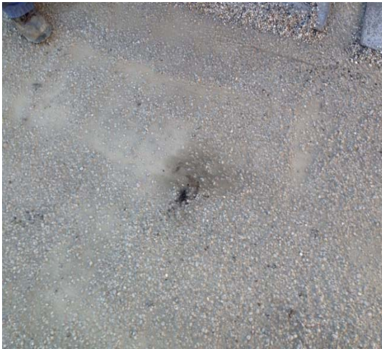
Current Condition of the Roof
