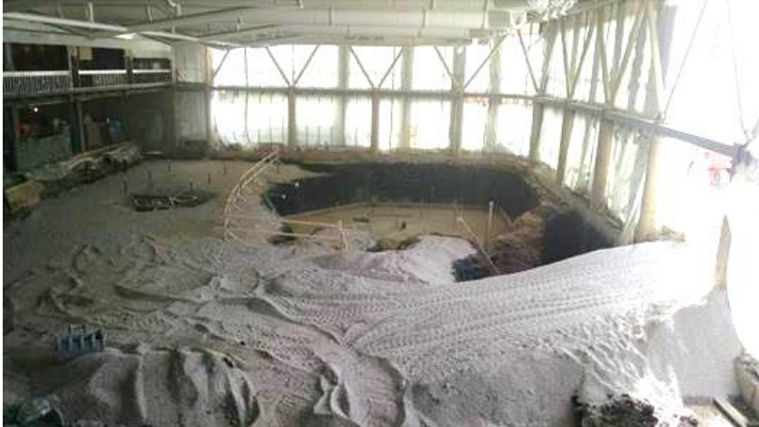
Progress Construction Photo showing pool area and diving well from March 2015
