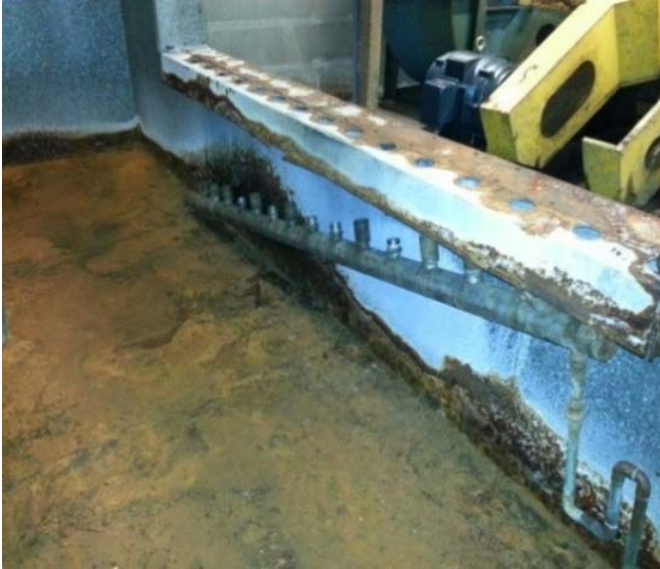
Current Condition of the Science Center Air Handlers.
