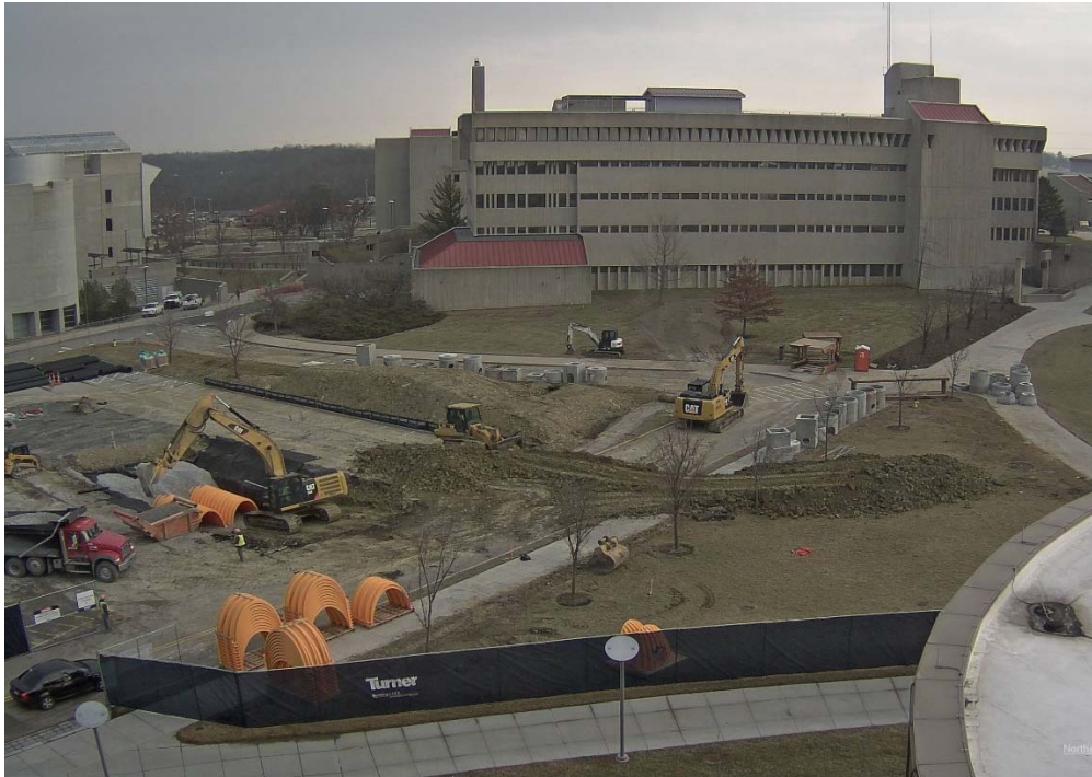
Construction Begins - Underground Utilities Being Installed
