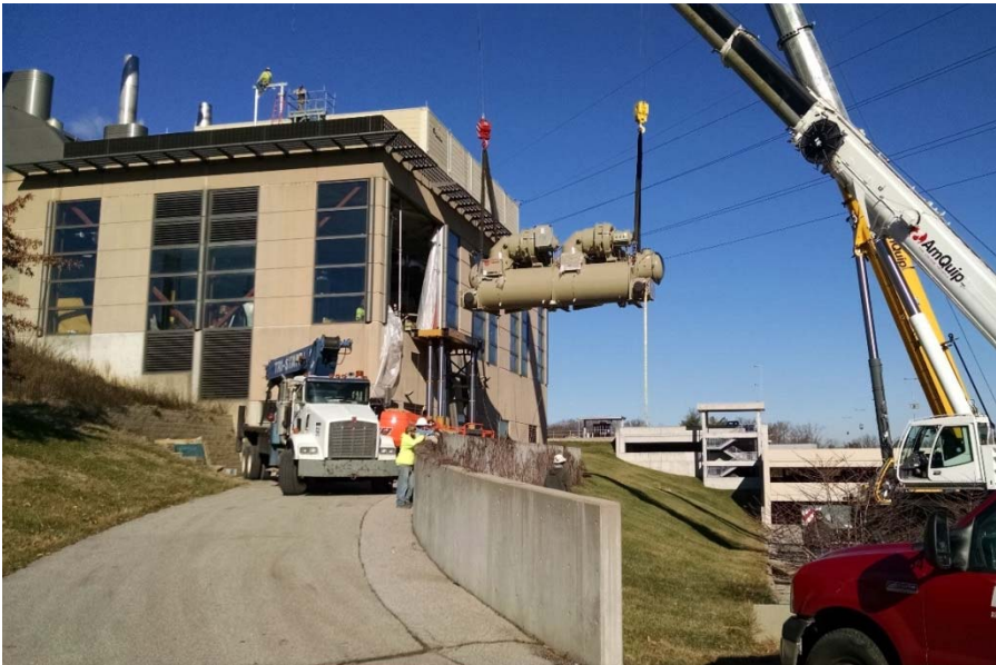
120,000 lb. Chiller being lifted into the Power Plant
