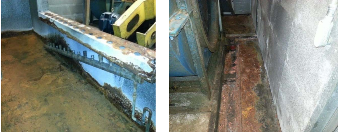
Current Condition of the Air Handlers and Mechanical Room
