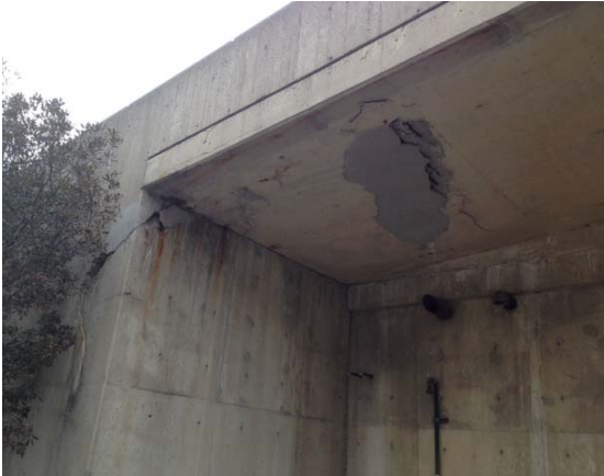
Current Condition of the Regents Hall/Student Union Bridge and the Stress Crack in the South Wall of Regents Hall
