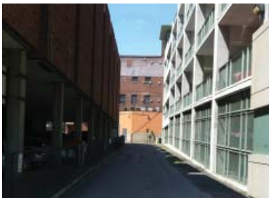
Above: Photos of existing GCTC Building
