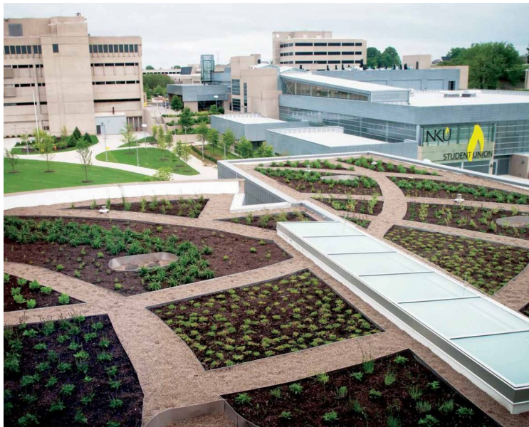
Griffin Hall Green Roof
