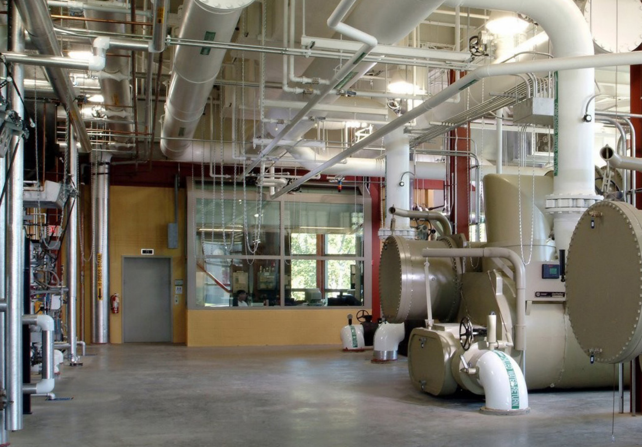
Central Plant / Photo credit: Champlin Architects
