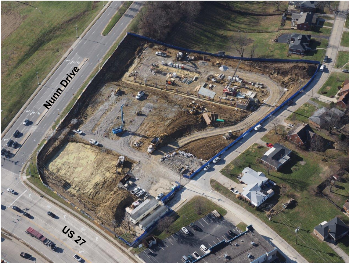
Aerial of Phase I Site as of January 4, 2019
